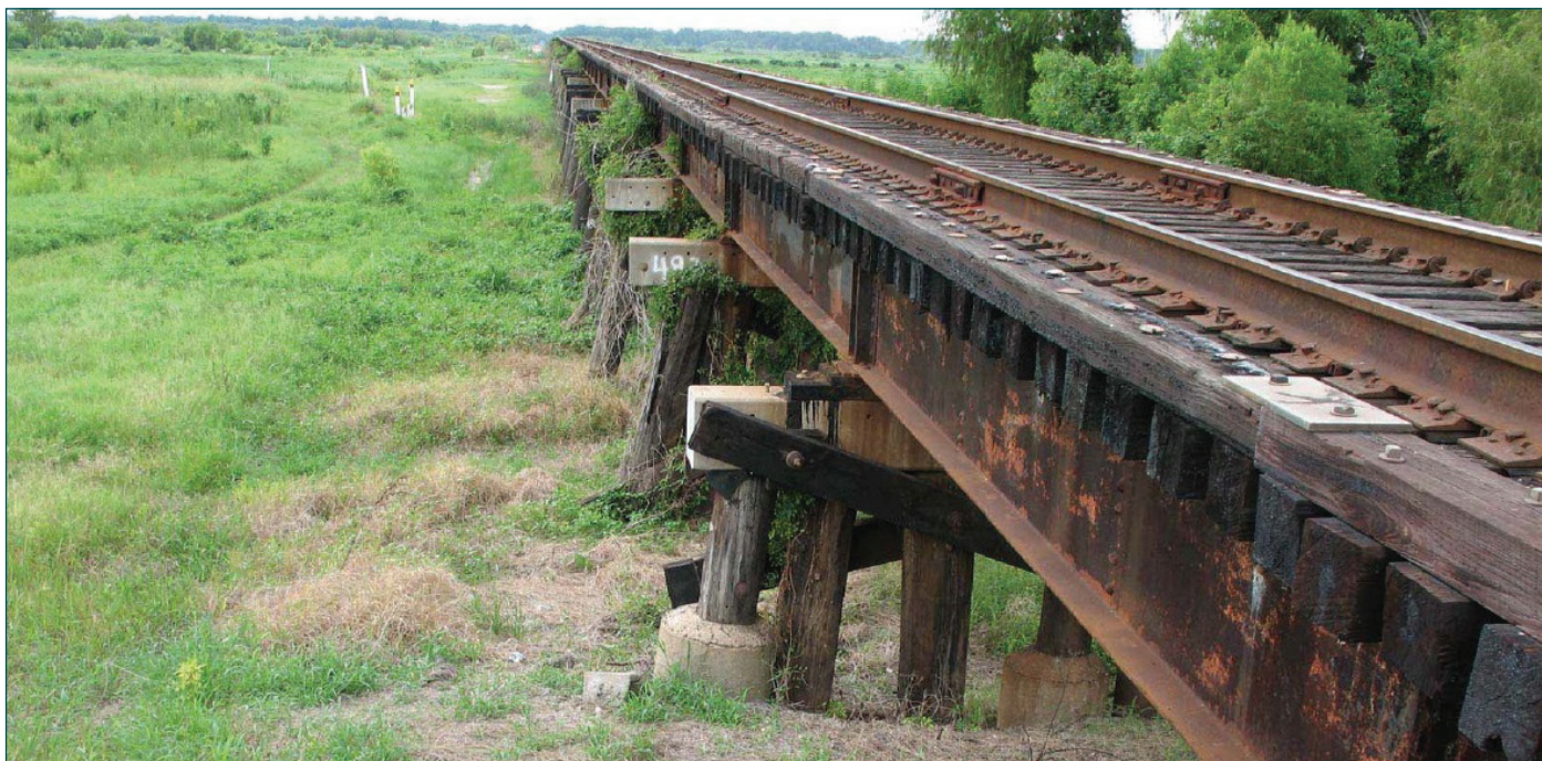
▲ Figure 8: The single track Bonnet Carré Spillway Bridge, with its 10 mph speed limit, is a major impediment to the growth of the freight traffic on the rail line.
